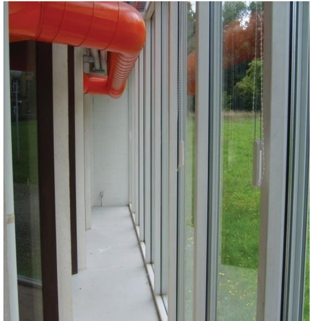
Figure 4. Buffer space with indirect gain.
