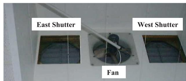
Figure 5. Heat extractor system.
